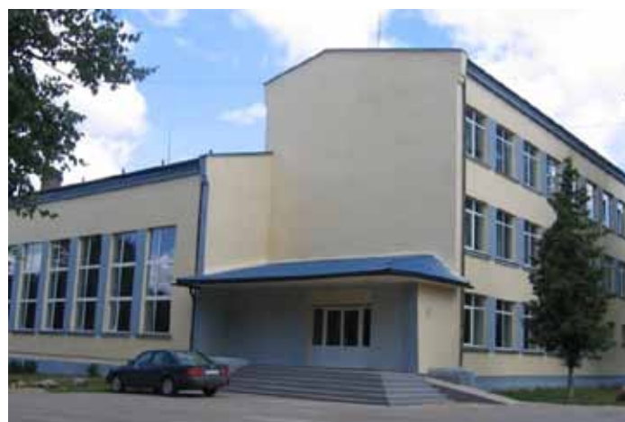
Fig. 6. Dagda culture house. Architects P. Švābe and E. Leitāne. 1959.
