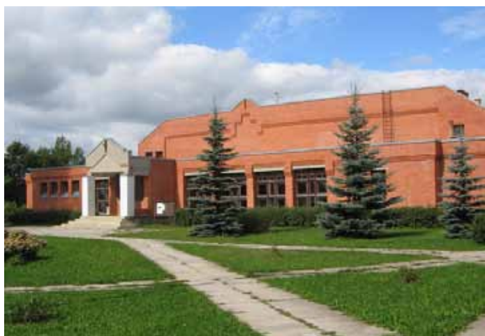
Fig. 19. The people's house in Pušmucova parish. 1989.
