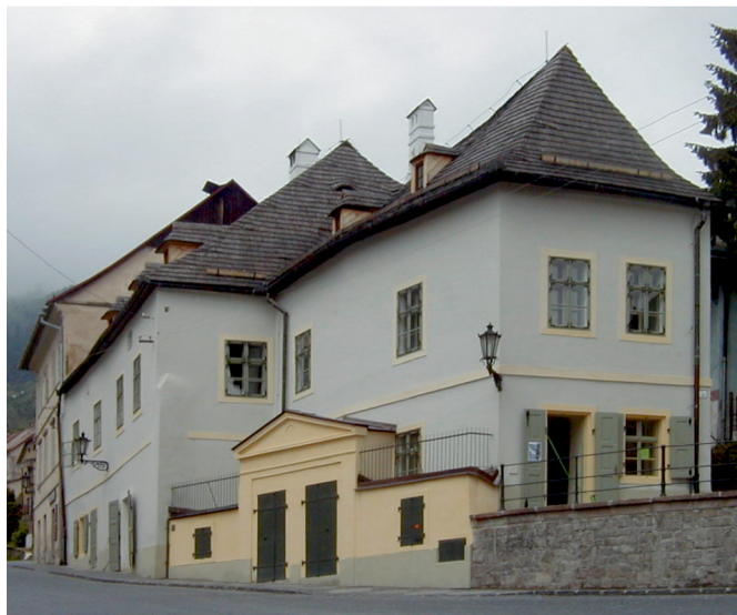
Fig. 2. Research and Education Center of the Faculty of Architecture in Banská Štiavnica, a place of experimental research and educational activities of national and international character.
