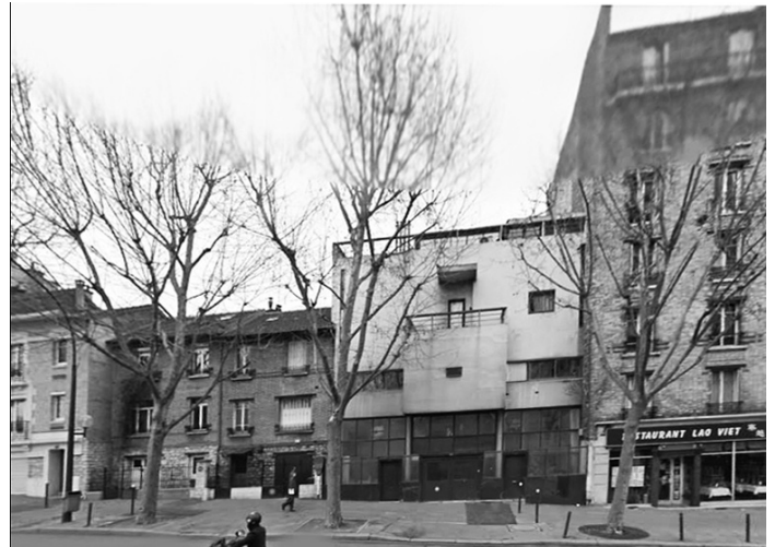
Fig. 3. Maison Planeix, Paris (1928). View from boulevard Massena [9]
