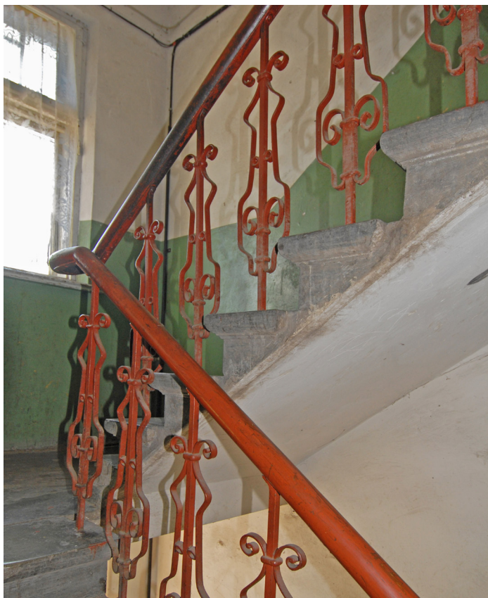
Fig. 29. Apartment house at Ferdinanda Grīniņa iela 3. A staircase
