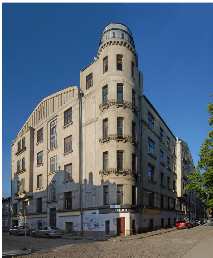
Fig. 11. Apartment house at Republikas iela 19. A view from the corner of Toma and Republikas Streets
