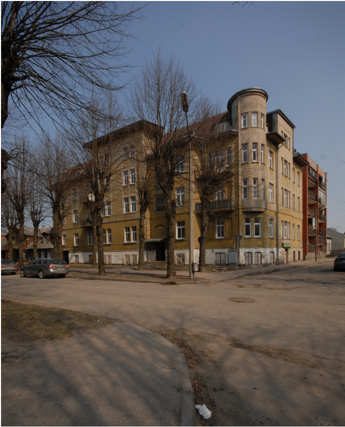
Fig. 14. Apartment house at Uliha iela 25. 1914
