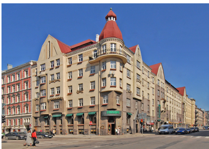
Fig. 34. Apartment house in Riga, at Aleksandra Čaka iela 55, 1910. A. Vanags and P. Kampe (?)
