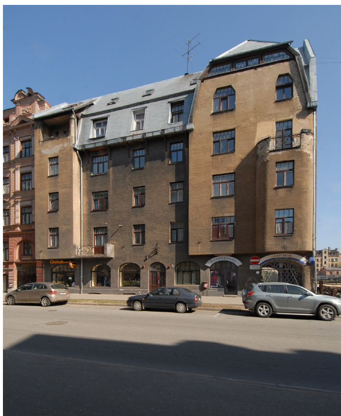
Fig. 6. Apartment house with shops in Riga, Ģertūdes iela 63. 1910. A. Schmaeling and P. Kampe (?)
