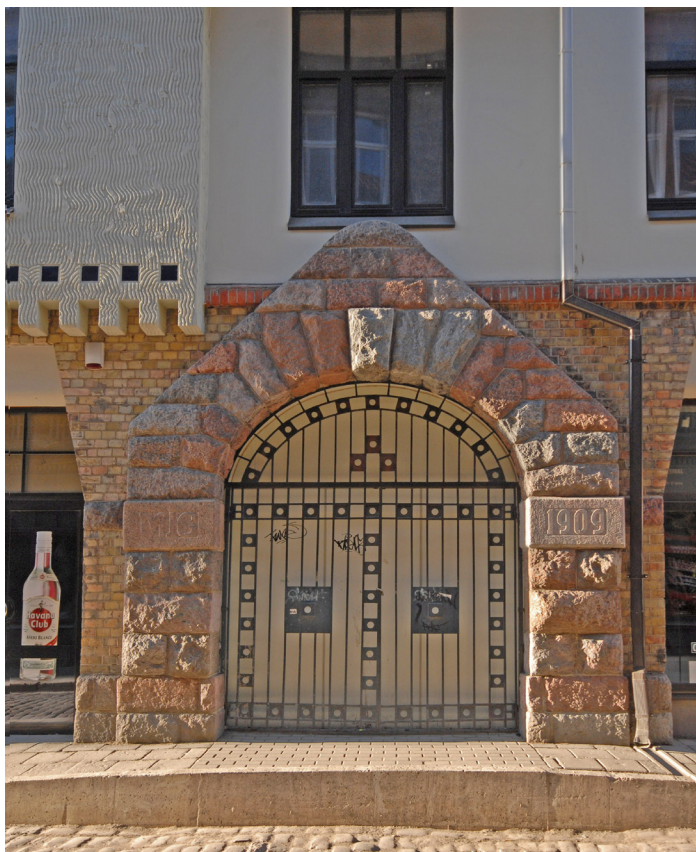
Fig. 35. Apartment house at Lielā iela 4. A portal on Pasta iela
