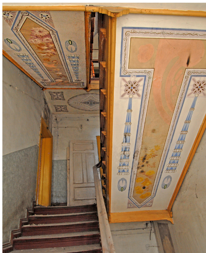
Fig. 38. Apartment house at Republikas iela 26/28. Finish details of the staircase
