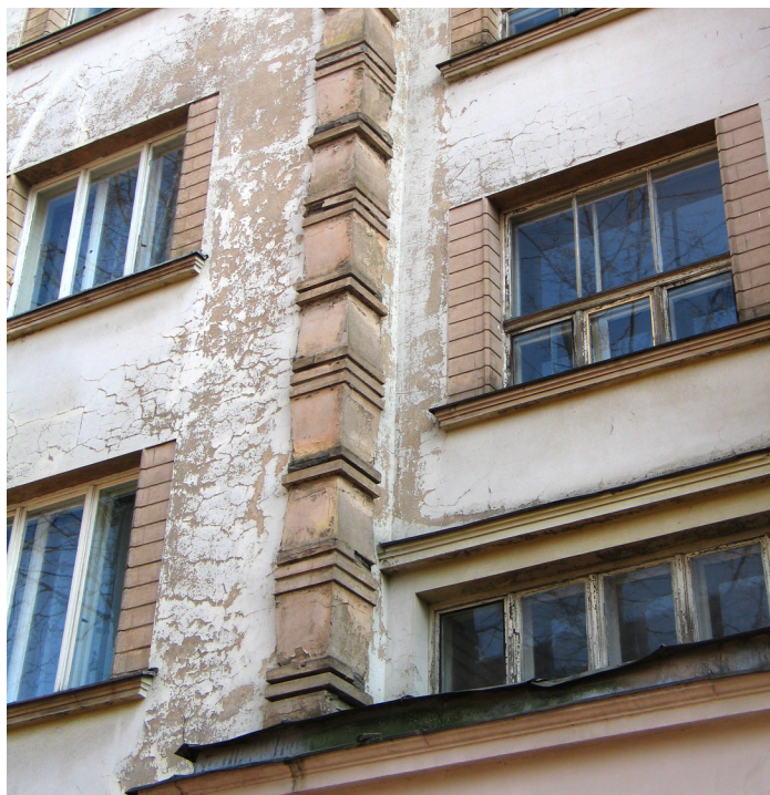
Fig. 26. Pauls Kundziņš, fragment of façade, apartment house at Tomsona iela 4, Riga, 1935 (Photo by Renāte Čaupale, 2009.–2012.)
