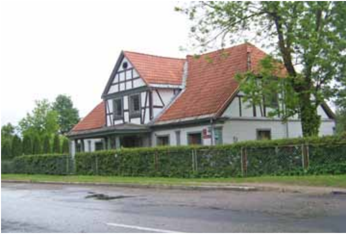
Fig. 3. The restored residential house at Dambja iela 17.
