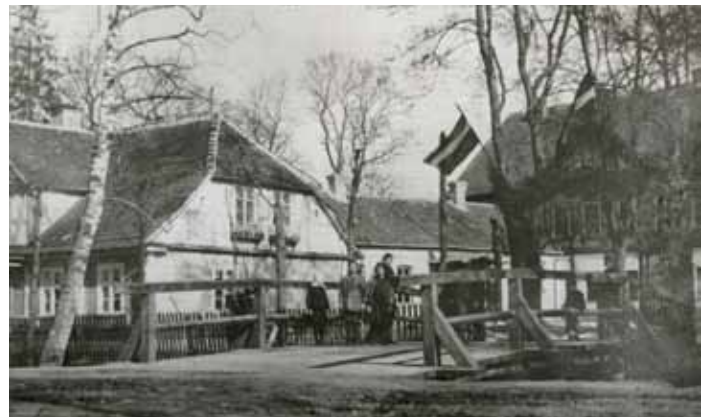
Fig. 1. The historical building along Duke Jacob's Canal (the 30s of the 20th century).
