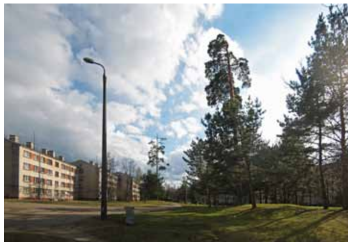
Fig. 12. Āgenskalna Priedes. Corridor-type buildings and a group of pine-trees at Kristapa Street.
