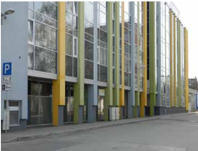
Fig. 13. Large-scale residential housing area courtyards in Riga, Rūpniecības iela, Riga, Latvia, 2012. [16]
