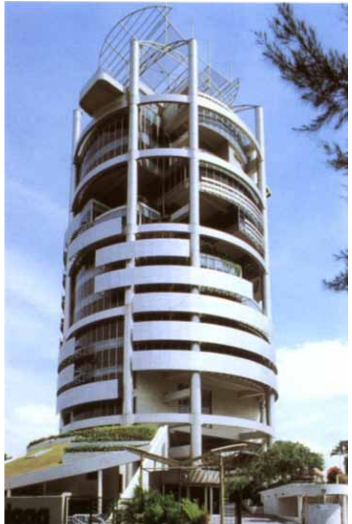
Fig. 8. The IBM headquarters in Kuala Lumpur, Malaysia. 1990-1992, K. Yeang. [9]
