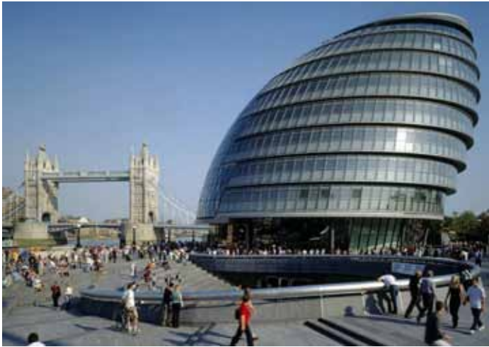
Fig. 9. City Hall in London, United Kingdom. 1998-2002, Foster and Partners [10].
