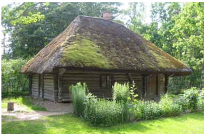
Fig. 1. A dwelling house from Vidzeme region. Open-air Museum, Riga, Latvia. A wooden log structure, compact in form with a low ceiling for heat retention. [Photo by the author]
