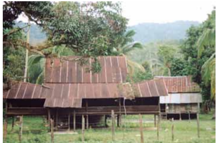
Fig. 2. A dwelling house. Negri Sembalan, Malaysia. The steep roof and the raised roof ends facilitate outflow of heated air from the rooms. [2]
