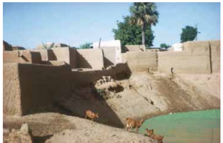
Fig. 3. A group of dwelling houses. Kano, Nigeria. The houses are built of earth, next to the place of excavation of the "building material". [2]
