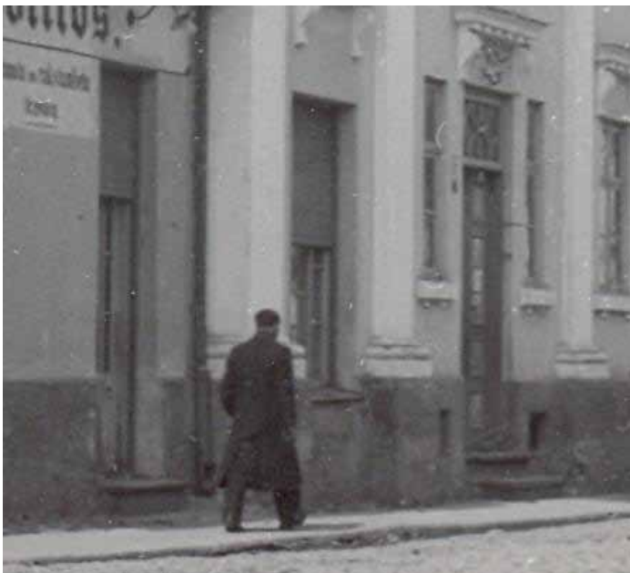
Fig. 5 and 6. Examples of implementation of Building Regulations in the 20s and 30s – Small roof with cantilevers on Kalna iela 22 [10] and steps at the building on Baznīcas iela 14 [11] have been countersunk in the aperture and with round corners.
