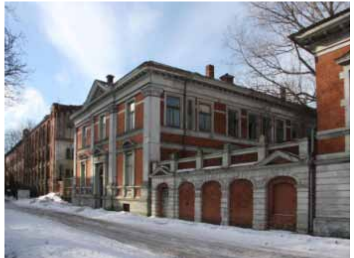
Fig. 29. Offices of linoleum factory of „Wicander & Larson”. Architect P. M. Bertschy. (Photo by Silvija Ozola, 2011).
