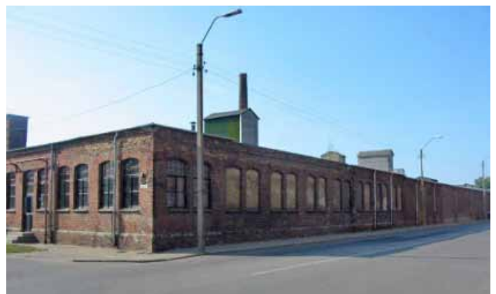
Fig. 36. Buildings along the perimeter of the oil factory „Kieler & Co” in Lazareva iela. Architect P. M. Bertschy. (Photo by Silvija Ozola, 2009)
