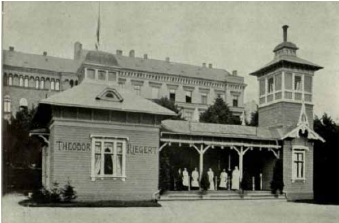
Fig. 6. The pavilion of Riegert's chocolate factory (architect R. Heuserman), 1901. [26]
