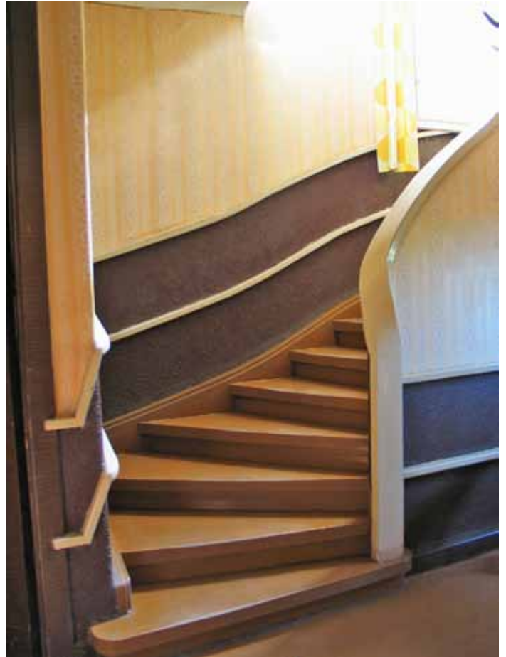
Fig. 15. Original colour scheme of living-room doors. Mansion at Strēlnieku iela 2, Ogre. 1935(?). Teodors Hermanovskis. [7].
