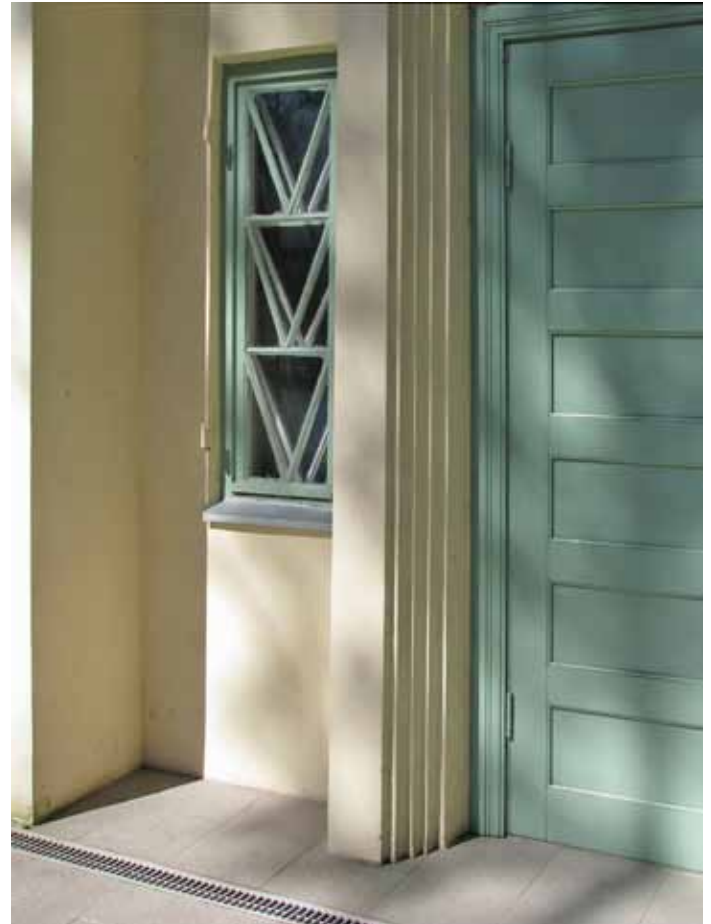
Fig. 4. Façade fragment. Mansion at Kalna prospekts 3, Ogre. 1927. Teodors Hermanovskis. [7]
