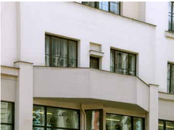
Fig. 6. Polygonal balcony, apartment and business house, Marijas iela (street) 8, Riga. 1926. Teodors Hermanovskis. [7]
