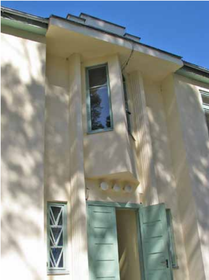
Fig. 2. Façade fragment. Mansion at Kalna prospekts 3, Ogre. 1927. Teodors Hermanovskis. [7]
